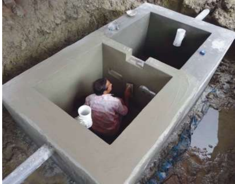
FIGURE 01: Two-chamber septic tank during construction. Source: Healthabitat.
