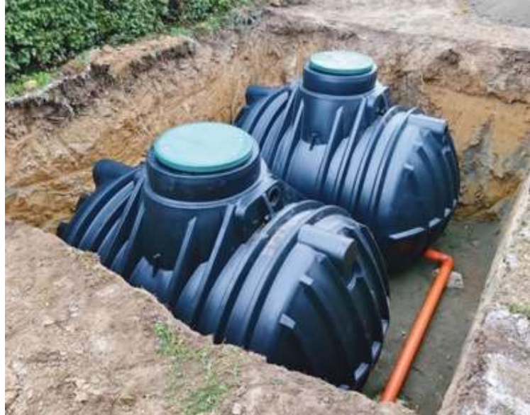
FIGURE 02: Prefabricated septic tank during underground installation. Source: Bowen's Septic Tank.
