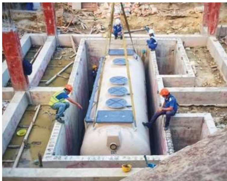
FIGURE 09: Johkasou Tank during installation. Source: Charm Limited.
