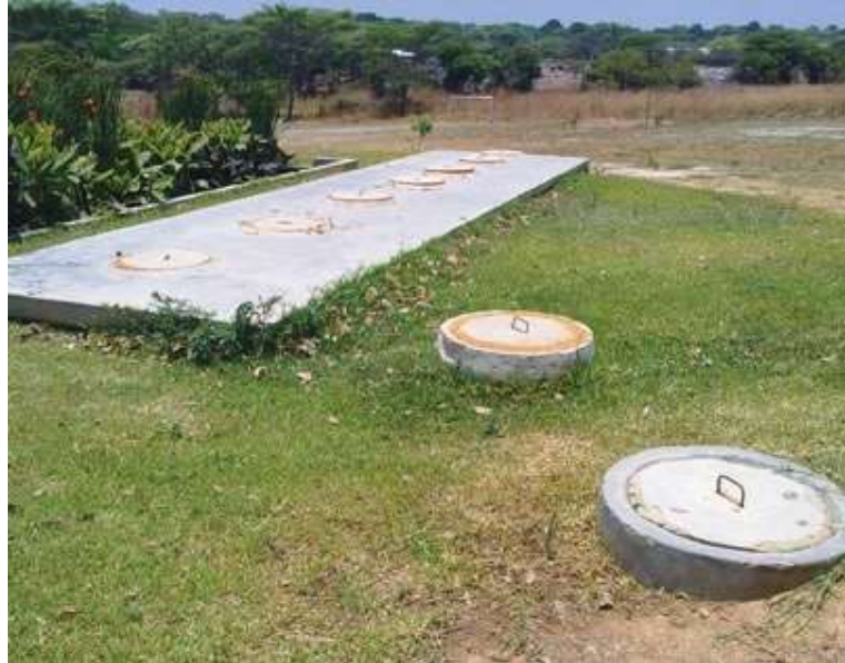
FIGURE 03: Installed ABR with manholes for each of the 6 chambers. Source: Gates Open Research, UPM, Anaerobic Baffled Reactor (ABR) Design Considerations for Faecal Sludge.
